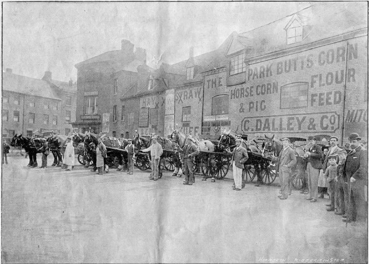
FRONT VIEW OF MR. CLEMENT DALLEY'S PARK BUTTS' ESTABLISHMENT.
