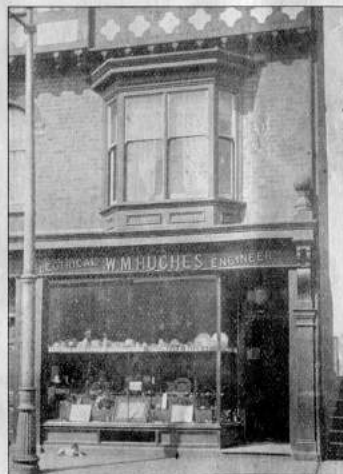
EXTERIOR OF Mr. W. M. HUGHES' SHOP
